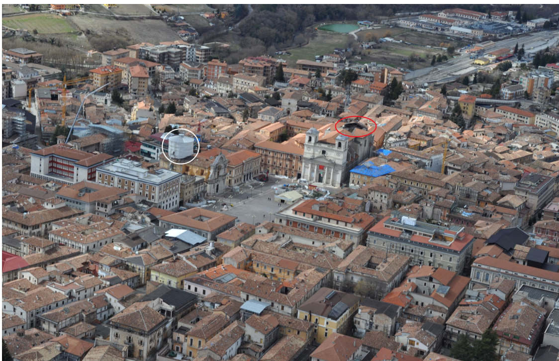
Figures 1 and 2. Above, a general view of the town of L'Aquila undergoing works of propping up and reinforcing buildings and provisional patching and waterproof covering of the roofs (blue, red or black) in March 2012. Below, a view of L'Aquila with "piazza del Duomo" in the center. Considerable damage (i.e. in the red oval) and conspicuous work of undergirding and securing (i.e. in the white circumference) of the churches, provisional patching and waterproof covering of the roofs (black or blue or red) and several cranes were evident in March 2012 at this geographical scale and other details become more clear with progressive zooms. Photos: Geographical Unit (Department of Documentary, Linguistic-Philological and Geographical Sciences) of the Sapienza University of Rome (in collaboration with GREAL, European University of Rome).
